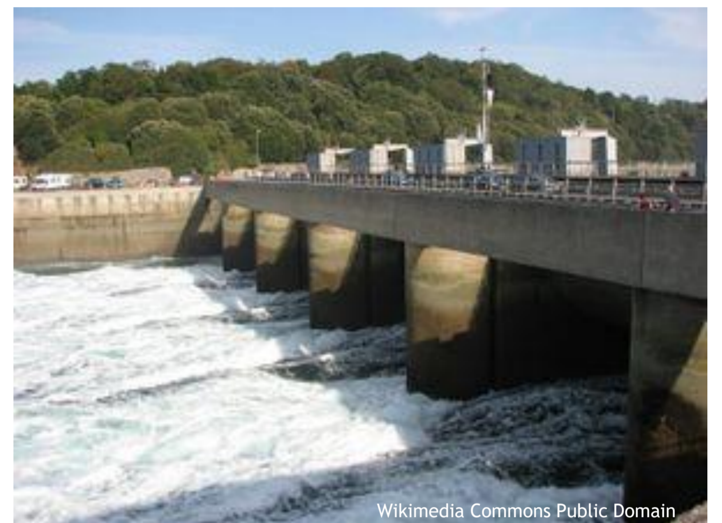
Dam of the tidal power plant on the estuary of the Rance River.
